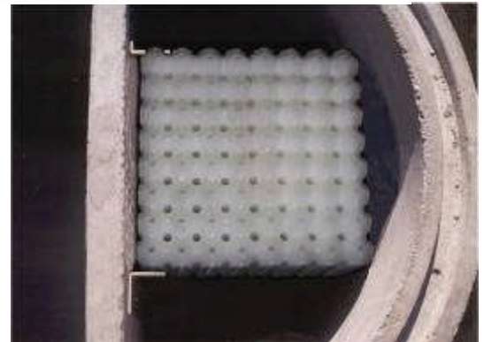
Modules installed in Manhole
